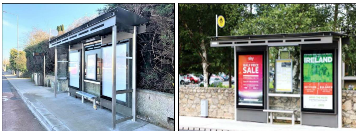
Figure 3.379: Example of a 3-Bay Reliance Cantilever Shelter with a Narrow Roof Configuration With and Without Half End Panels (Source: PDG)
