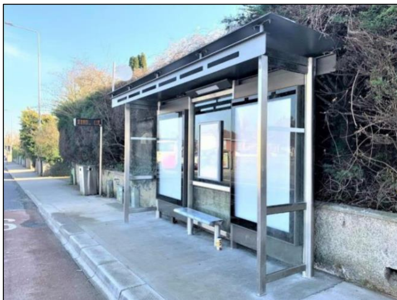
Figure 3.375: Example of a 3-Bay Reliance Cantilever Shelter with a Narrow Roof Configuration With and With Half End Panels (Source: PDG)
